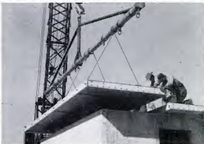
Above, workman is welding a corner joint in the upright walls. The walls are also welded to steel base plates set in the concrete pier-type foundations. Below, as roof panel is lowered by crane, two men ease it into proper position. These roof slabs are six inches thick and are welded to the walls and to each other to form a sturdy home.
